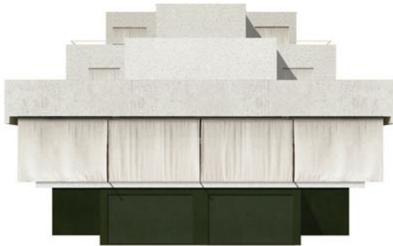
Residential building - Oberwil
